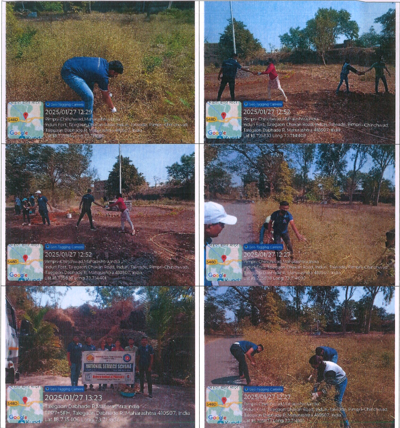
NSS Volunteers of MCOP Nigdi doing the FORT CONSERVATION On 27/01/2025
